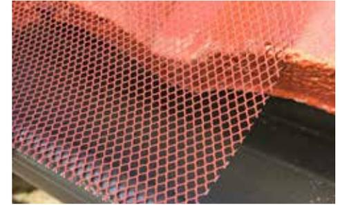
**STEP 1.** Place the roll of mesh on the roof with the edge of the mesh facing the gutter. The edge of the mesh should rest on top – and just inside – the edge of the gutter.
