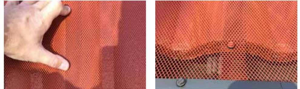
**JOINING MESH** When joining two pieces of mesh, overlap the mesh by 20mm. Place a metal screw through the centre of the overlap.
