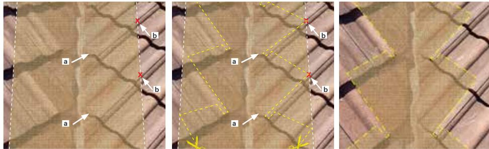
**STEP 3.** Using tin snips, cut the mesh on either side of the valley using points (a) and (b) as a guide. The notches (approximate thickness of the tile) created at point (a) will allow the mesh to transition from above to below the tile easily.
