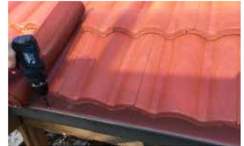
**STEP 2.** Roll the mesh out along the gutter edge.
