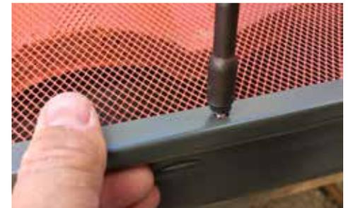
**STEP 3.** Place the standard or Mesh Lock trim over the mesh. The mesh should rest under and against the front edge of the trim. Secure by placing a metal screw in every pre-made hole. Do not over tighten the metal screws.
