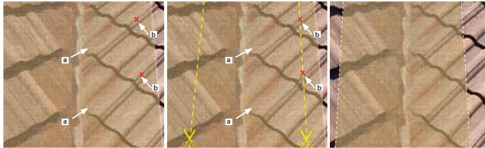
**STEP 2.** Determine two points up the valley where the mesh will transition from over the tile to under the tile (a), and length of the flap which will be tucked under the tile (b), all the way up the valley on each side. Using tin snips trim the excess mesh away where these two points intersect up the valley on each side.
