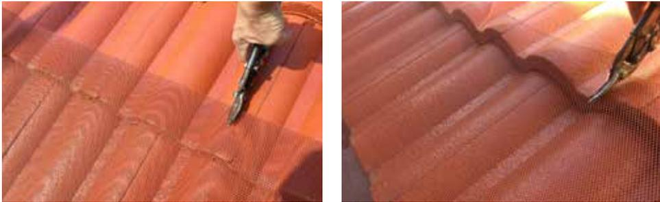
**STEP 4.** Using offset tin snips, cut a slit in the back of the mesh next to the overlap in every tile.
