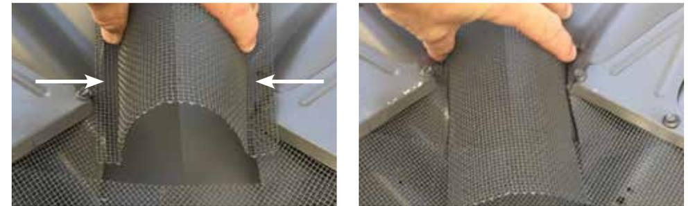
**STEP 2.** To fit the domed valley mesh, squeeze the mesh together until the folded edges fit beneath the roof sheet on both sides of the valley. Release the mesh so that it spreads and fits snugly under both edges of the roof.
