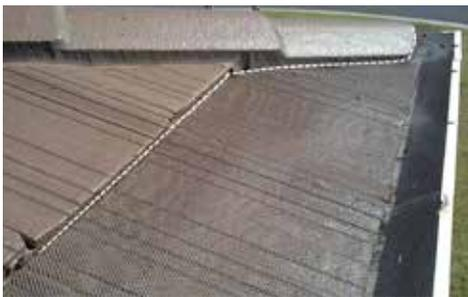
**STEP 6.** If the hips and gable ends are secure with concrete, you will be unable to lift the second tile. Instead, cut the mesh to be in line with the front of the second row of tiles and seal with silicone (if required).
