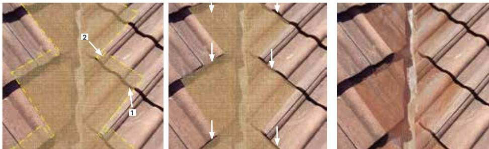
**STEP 4.** Using a flat head screw driver, lever the upper tile off the lower tile (1) and then tuck each flap created previously (2) under, before lowering the tile back in place. Press down firmly to lock the mesh into position being careful not to damage the tile.
