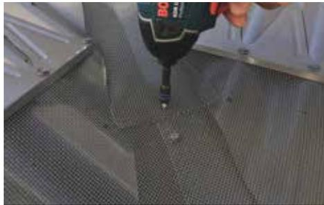
**STEP 5.** Secure each overlapping section of valley mesh together using metal screws provided. For narrower valley mesh, one screw per join is sufficient. For wider mesh, use two screws.
