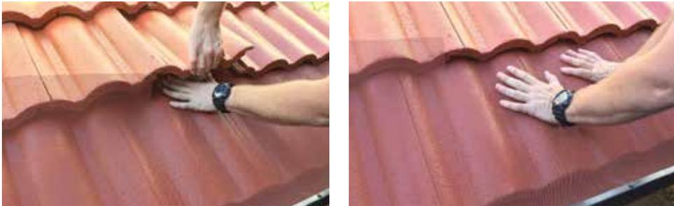
**STEP 5.** Tuck the mesh under the tile by lifting the second row of tiles from under the mesh. Use a flat head screwdriver to lever the second tile up as required.
