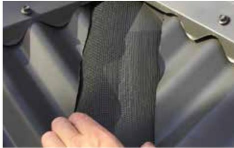
**STEP 4.** Start fitting the domed valley mesh at the bottom of the valley, 100mm up from the end of the roof sheet where it enters the gutter. Work up to the ridge overlapping each section by 4 mesh squares. The valley mesh should be fitted over the top of the regular gutter mesh at the bottom of the valley.
