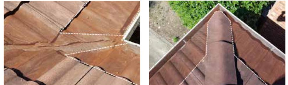
**CORNERS** Cut the mesh around the edge of the ridge capping. Overlap the mesh above the gutter and join using a metal screw.
