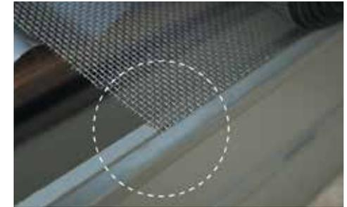
**STEP 1.** Place the roll of mesh on the roof with the cut edge of the mesh facing the gutter. The cut edge of the mesh should rest on top – and just inside – the edge of the gutter.
