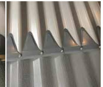
**STEP 8.** Screw to the roof sheet and continue along mesh length.
