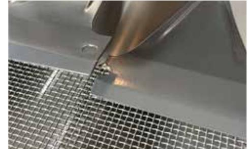
**STEP 7.** Overlap the profiles by placing the closed end screw hole over the open end screw hole.
