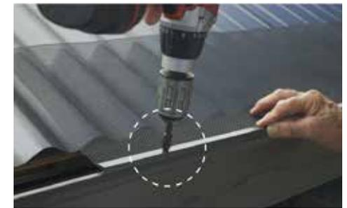
**STEP 3.** If standard or Mesh Lock trim is used, place the metal trim over the mesh. The mesh should rest under and against the front edge of the trim. Secure by placing a metal screw in every pre-made hole. Do not overtighten the metal screws.
