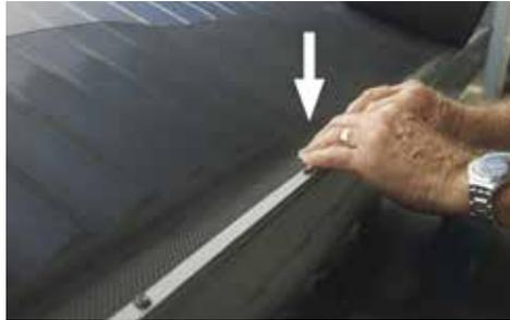
**STEP 4.** For 2mm mesh, pinch the mesh at the gutter edge to form a horizontal platform. This will create a water break to prevent water from flowing to the edge of the mesh during heavy rainfall. For 4mm or 5.4mm mesh, you should consider pinching the mesh when the roof pitch is steep (over approx, 30°)
