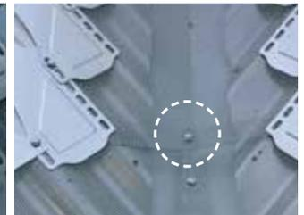
**STEP 4.** Screw the multi-pitch fins to the roof sheet ensuring the screw penetrates through the mesh below. Do not overtighten the metal screws.
