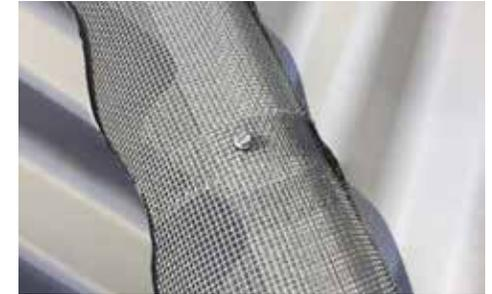
**STEP 4.** Secure each overlapping section of valley mesh together using metal screws provided. For narrower valley mesh, one screw per join is sufficient. For wider mesh, use two screws.
