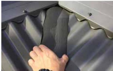
**STEP 3.** Start fitting the domed valley mesh at the bottom of the valley, 100mm up from the end of the roof sheet where it enters the gutter. Work up to the ridge overlapping each section by 4 mesh squares. The valley mesh should be fitted over the top of the regular gutter mesh at the bottom of the valley.
