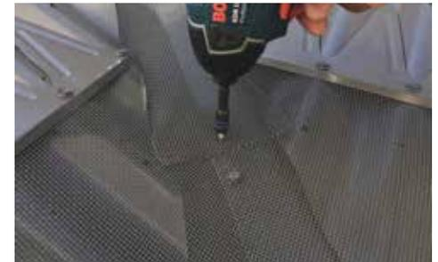
**STEP 5.** Push the dome flat at the top and bottom to close off all openings and secure the lap with metal screws.
