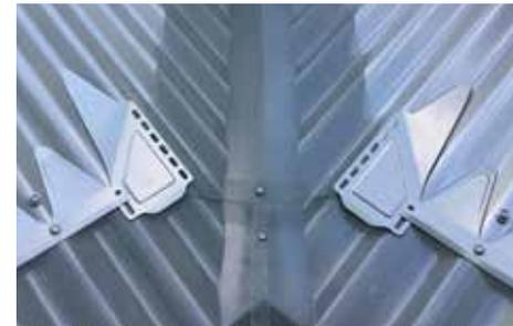
**STEP 2.** Place No.1 & No.2 multi-pitch fins over the mesh and on either side of the valley. Looking up the valley from the gutters internal corner, typically the No.1 multi-pitch fins are placed on the right and No.2 multi-pitch fins on the left.
