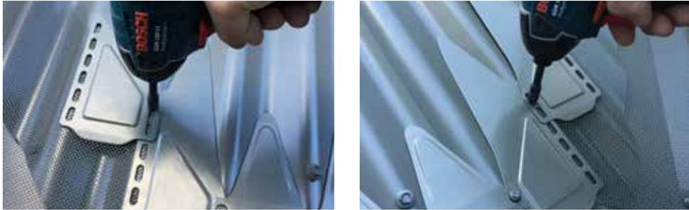
**STEP 4.** Screw the multi-pitch fins to the roof sheet ensuring the screw penetrates through the mesh below. Do not overtighten the metal screws.
