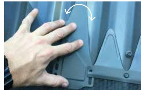
**STEP 3.** Move the first multi-pitch fins from left to right finding the ideal fit within the roof contour.
