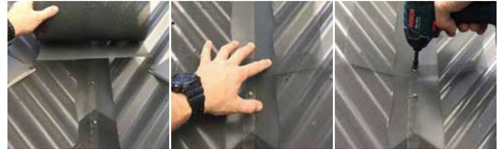
**STEP 1.** Roll the required length of mesh along the valley gutter, overlapping the gutter mesh by 20mm at the centre of the valley. Valley mesh should be installed last to ensure it sits on top of the gutter mesh at the gutter.
