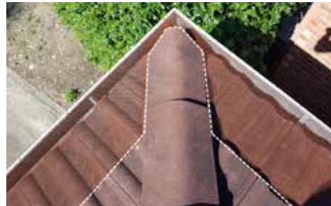
CORNERS Cut the mesh around the edge of the ridge capping. Overlap the mesh above the gutter and join using a metal screw.
