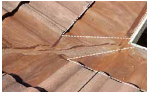
CORNERS Cut the mesh around the edge of the ridge capping. Overlap the mesh above the gutter and join using a metal screw.
