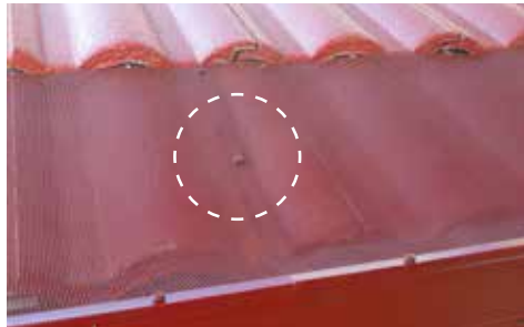
JOINING MESH When joining two pieces of mesh, overlap the mesh by 20mm. Place a metal screw through the top and centre of the overlap.
