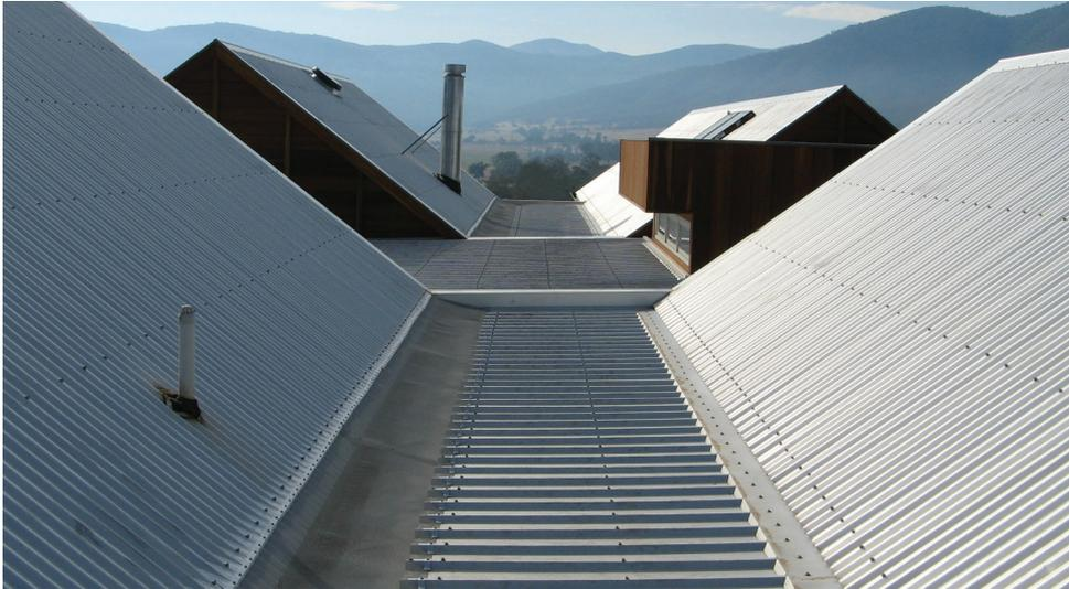
Box gutters are typically positioned within the body of a roof and not visible from the ground. They are typically boxed in on all sides between roof sheets, or behind parapet walls.
