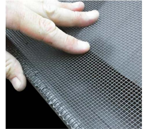
**STEP 1.** Place the roll of mesh on the roof. The edge of the mesh should rest on top – and just inside – the gutter edge.
