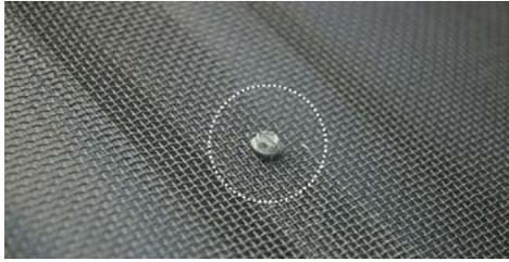
**JOINING MESH.** When joining two pieces of mesh, overlap the mesh 20mm. Place one screw through the centre of the overlap.
