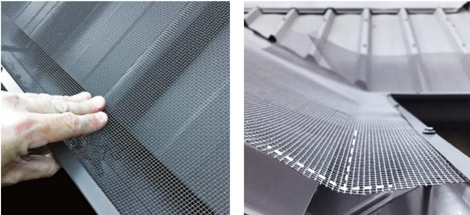
**STEP 4.** For 2mm mesh, pinch the mesh at the gutter edge to form a horizontal platform. This will create a water break to prevent water from flowing to the edge of the mesh during heavy rainfall. For 4mm mesh, you should consider pinching the mesh when the roof pitch is steep (over approx. 30°).
