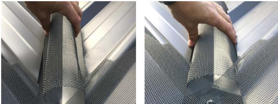
**STEP 1.** To fit the domed valley mesh, squeeze the mesh together until the folded edges fit beneath the roof sheet on both sides of the valley. Release the mesh so that it spreads and fits snugly under both edges of the roof.
