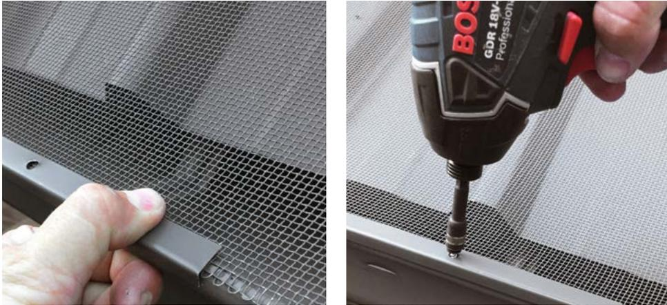
**STEP 3.** Place the standard or Mesh Lock trim over the mesh. The mesh should rest under and against the front edge of the trim. Secure by placing a metal screw in every pre-made hole. If trim is not used, screw the mesh to the gutter edge every 250mm.
