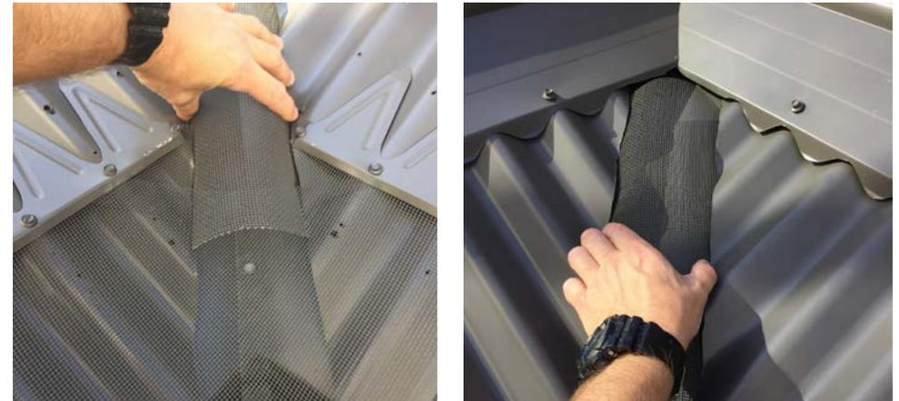
**STEP 3.** Start fitting the domed valley mesh at the bottom of the valley, 100mm up from the end of the roof sheet where it enters the gutter. Work up to the ridge overlapping each section by 4 mesh squares. The valley mesh should be fitted over the top of the regular gutter mesh at the bottom of the valley.
